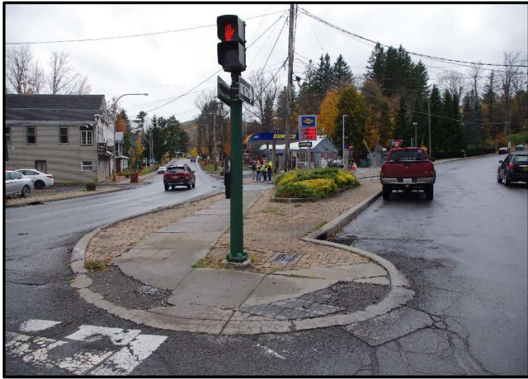
2020 – Existing sidewalk condition in Village
